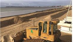
Fig. 4. Work for the creation of the Ecoplage, on the beach of La Baule, january 2019.
